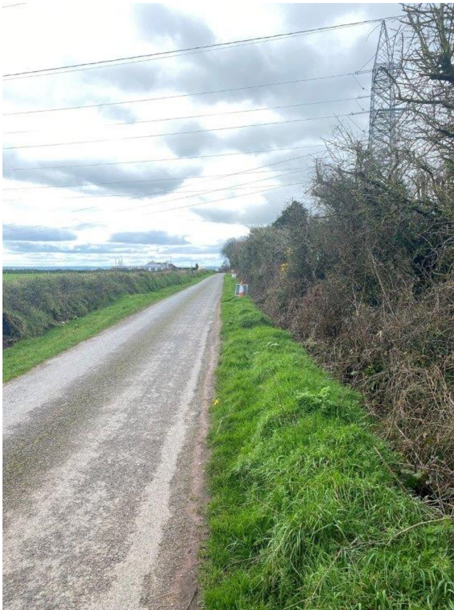
Image 9: Proposed cable route location along the L6989 to the south of the existing 220kV substation site
