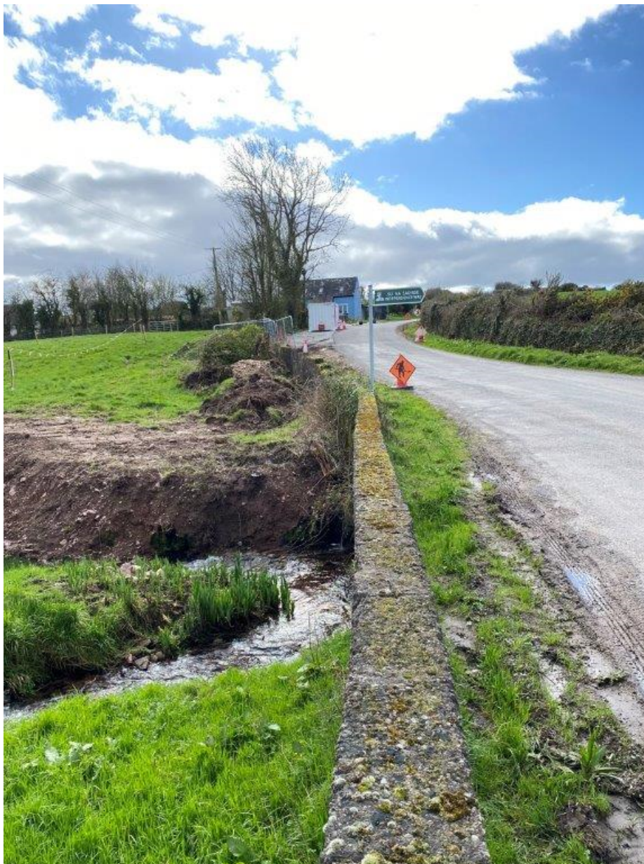
Image 10: Existing bridge along the L6989 spanning the Butlerstown River tributary (approximately 615m east of the proposed site)
