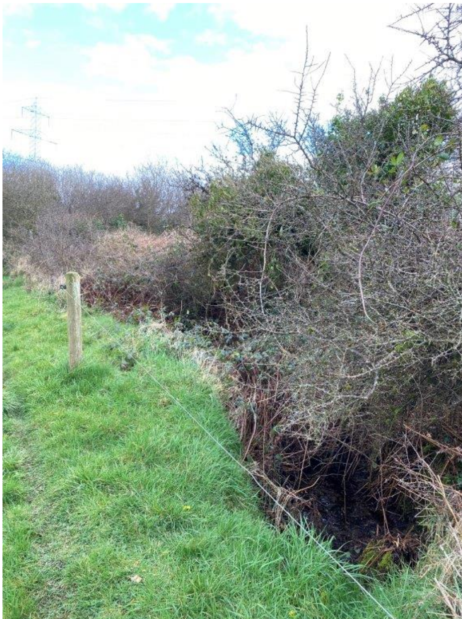
Image 8: Drainage ditch along southern boundary of proposed substation site
